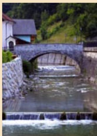
Most pod Grivo Bridge
